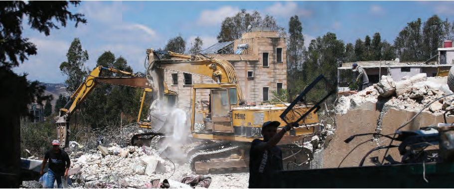
Residents clear rubble from their homes destroyed during the Israel-Hezbollah war in Ghandouriyeh village, southern Lebanon on Tuesday
